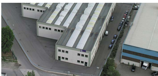
Pian Camuno (Bs - Italy) electrical equipment
