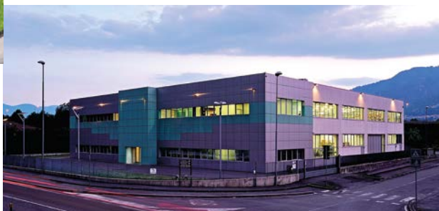
Pisogne (Bs - Italy) level, pressure, temperature sensors
